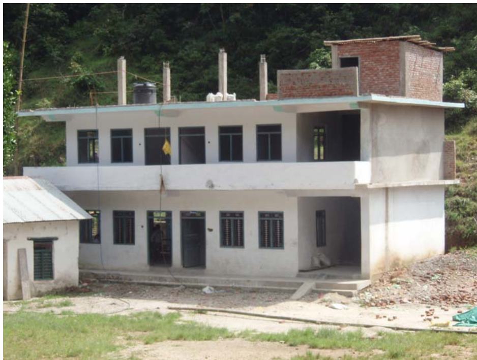
Newly constructed building
